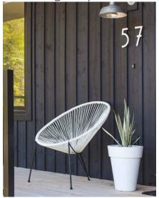
Evolution Series is the next generation of siding; combining tongue & groove, end-matching, hidden nail and modern design. Fraser Evolution Series makes installation a breeze by locking in every board on all four sides; top, bottom and both sides. End-to-end siding joints no longer need to end on strapping/furring/studs. The hidden nail system provides a cleaner look by virtually eliminating
